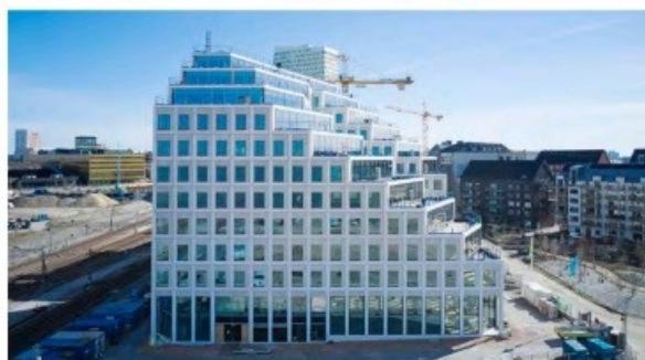
Hyllie Terrass, a climate neutral building in white concrete. Façade claddings produced by UPB Group based on Aalborg White cement.
