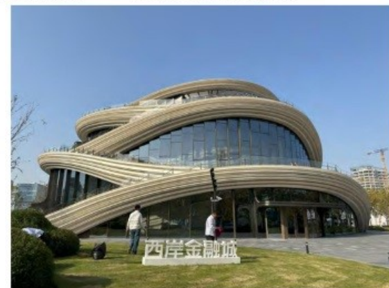
Shanghai West Bund Orbit designed by Heatherwick studio, using Aalborg White cement based GRC Claddings.
